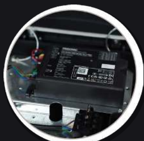
Driver compartment — removable wiring plate
